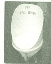
Chris Melo traded his boat's holding tank for a urine-diverting composting toilet and a self-made urinal, Mr. PeeBuddy. He pours urine into a rain barrel that flows to drip-irrigation lines in his garden.
