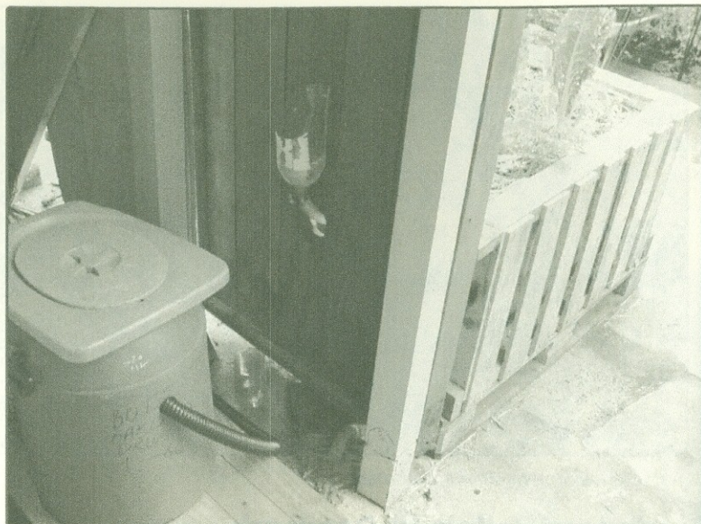
The outdoor toilet and urinal at City Slicker Farm. The urinal drains directly to a planter growing leafy greens.
